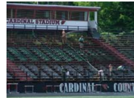
Home Bleacher Demolition 5/07
