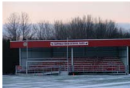
Band Shell Construction 10/06
