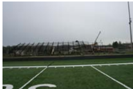
Visitor Bleacher Demolition 1/07
